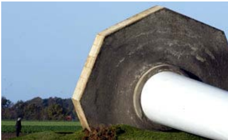
Figure 15. A 70-meter or 230-foot high tower collapsed in inclement weather at Goldenstedt, Germany, on October 28, 2002.
