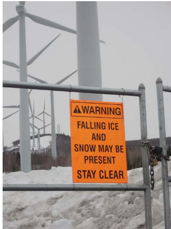
Figure 29. Judicious warning about ice shedding and limited access at a wind turbine site, USA.
