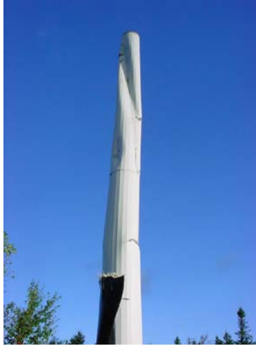
Figure 9. Turbine collapse in high wind conditions at the Searsburg, Vermont wind facility, September 15, 2008.
