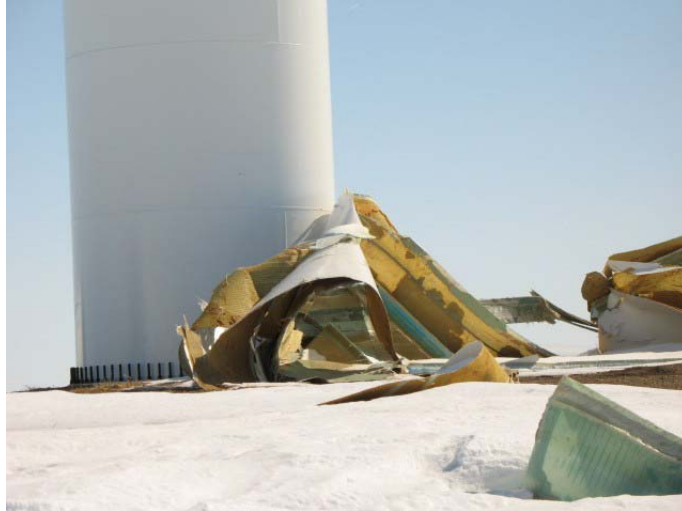
Figure 17. Turbine failure at Lake Wison, Minnesota, November 2007.
