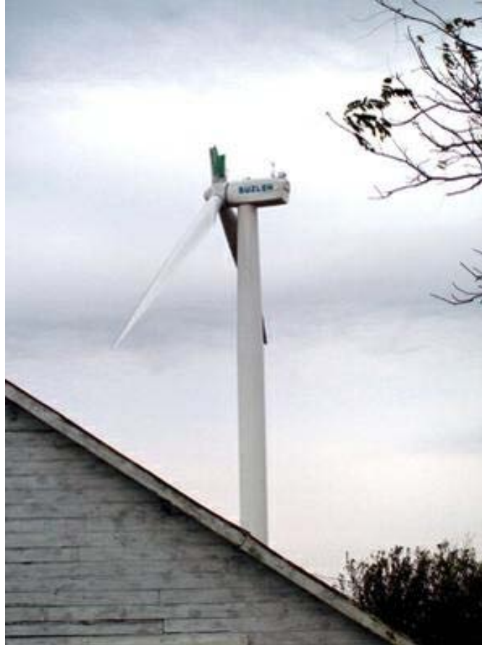
Figure 16. Blade failure at the stem on a 140 feet radius wind turbine at Wyanet, Bureau County, Illinois, October 22, 2008. The blade landed 150 feet from the base of the structural tower.
