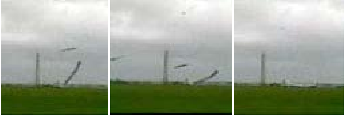
Figure 11. Runaway turbine disintegration clip sequence from video caused by failure of brake system, 2008. Notice how an initiating event of a single blade failure evolved into a failure sequence where the unbalanced nacelle and hub caused another failed blade to hit the structural tower, slicing it and causing it to collapse while the disintegrated rotor blades were ejected away. Source: UTube.
