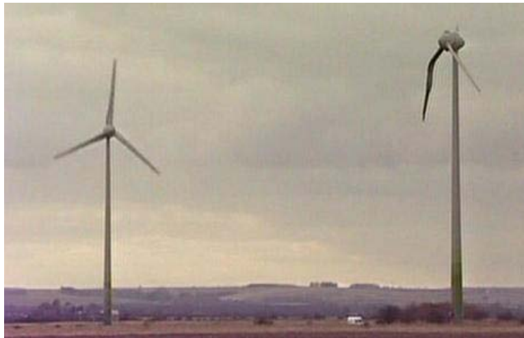
Figure 27. Blade failure due to possible ice shedding from one blade unto another or a manufacturing defect, Conisholme, Lincolnshire, UK.
